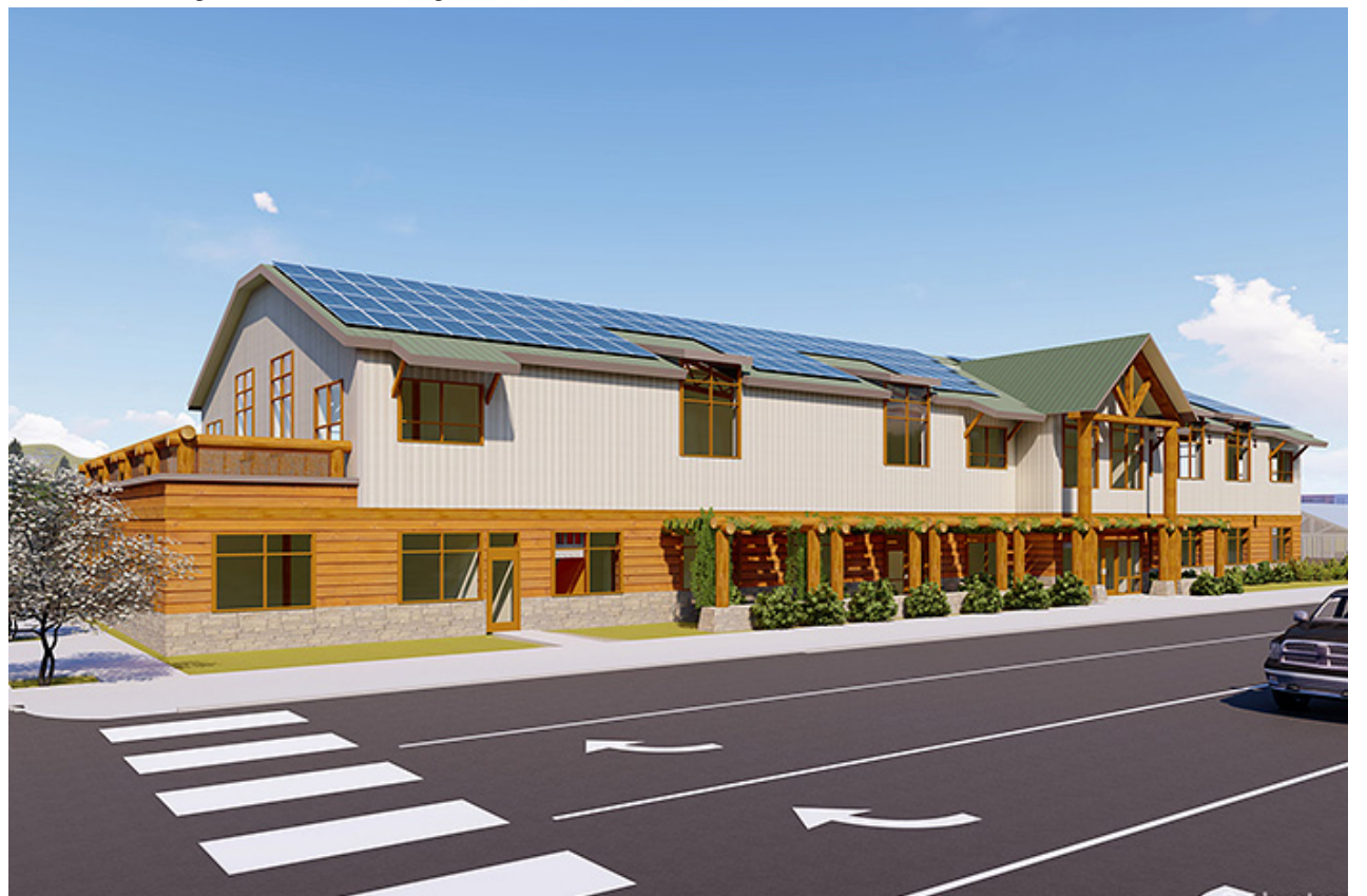
Oregon State University’s Extension Service Education Center is expected to have net-zero energy consumption, thanks in part to a rooftop photovoltaic array. (Courtesy of Soderstrom Architects)
